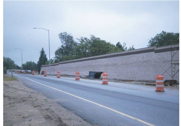
US 36 and Federal Blvd Post-Tensioned Masonry Soundwall
