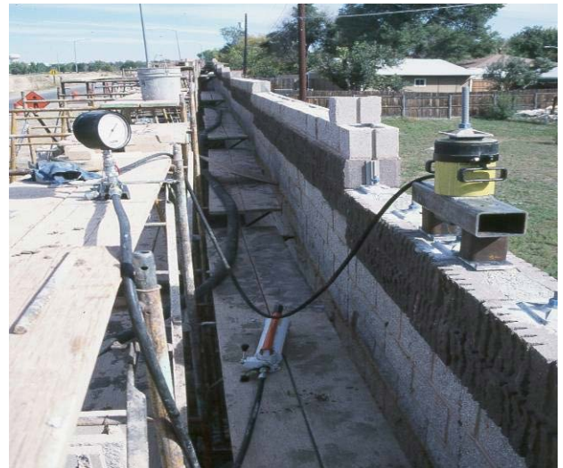
Hydraulic pump and ram used to tension the intermediate tendons.
