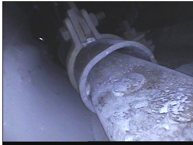
Videoscope image of interior armature and attachment point with plinth at bronze rivet heads.
