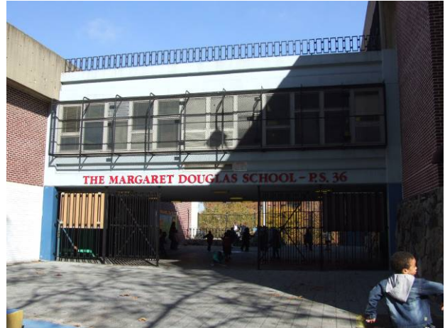
Overall view of school entrance
