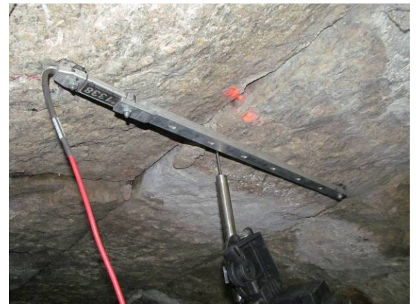
Instrumentation used to measure displacements and strains
