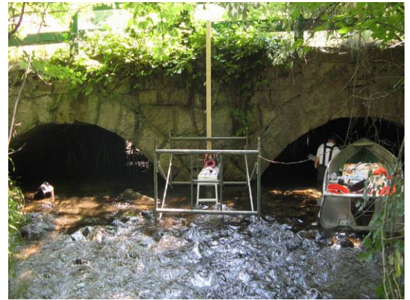
Two-span masonry arch bridge located in Burrillville, RI
