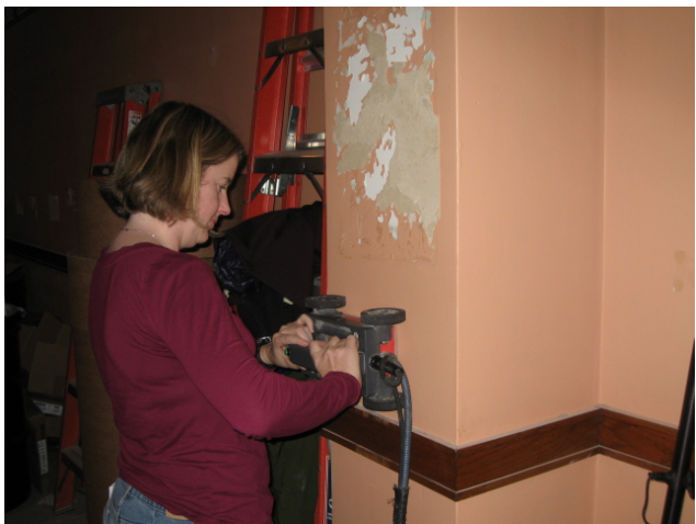
Examining embedded steel columns with radar
