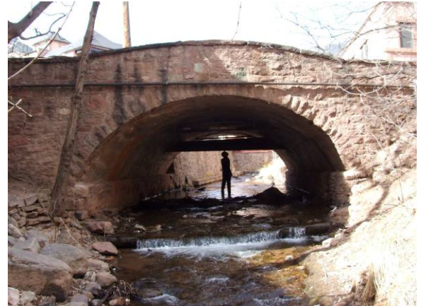
Canyon Ave Bridge
