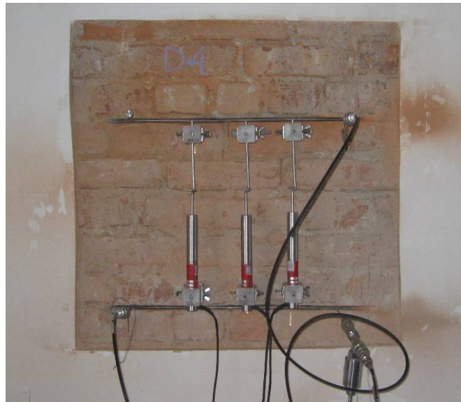
On-site flatjack deformability test
