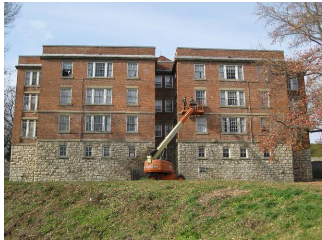
Building 427 located in Ft. Leavenworth, KS
