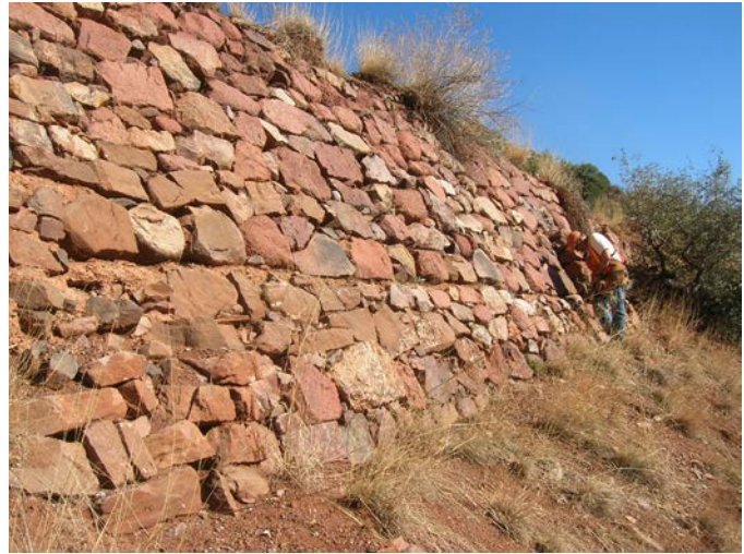
Typical stone masonry walls along the Coronado Trail
