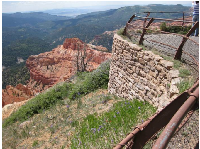
Stone masonry retaining wall at Chessman Overlook, UT
