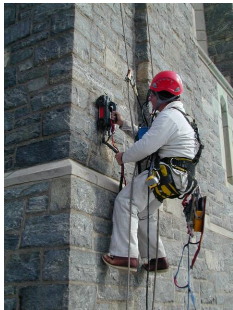
Scanning with radar for bond stones
