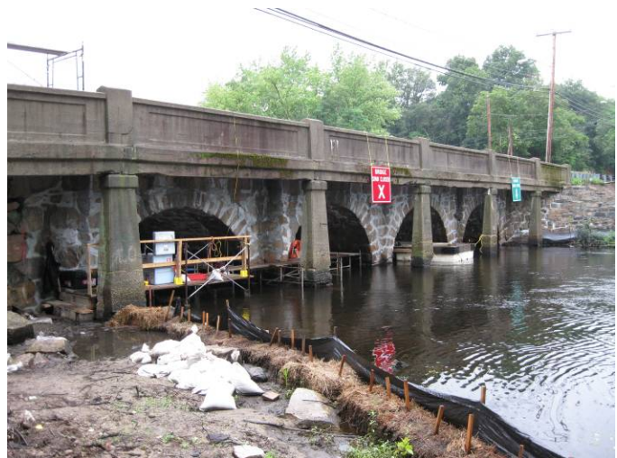
Four-span masonry arch bridge located in Dedham, MA
